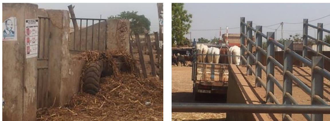
Fig. 5.– Examples of well-maintained and poorly maintained livestock loading and off-loading chutes
